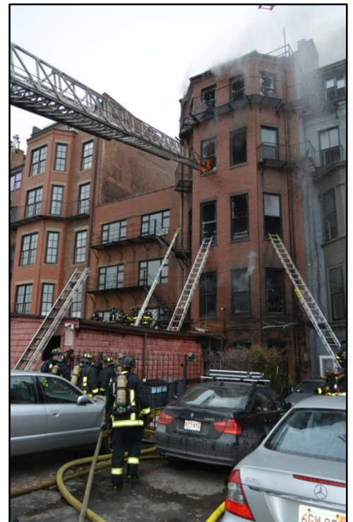
A view of fireground from Side Charlie. The fire started near the one-story shed (located against the fence) and extended into hallway on the basement of the structure.
