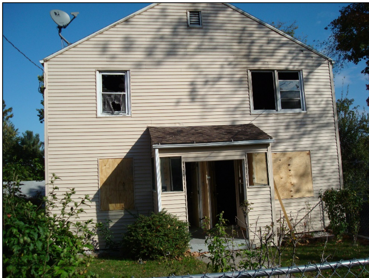
Photo 1. Side Alpha—street view of the duplex. Engine 16 and Ladder 4 made entry into the building through the left doorway. (NIOSH photo.)
