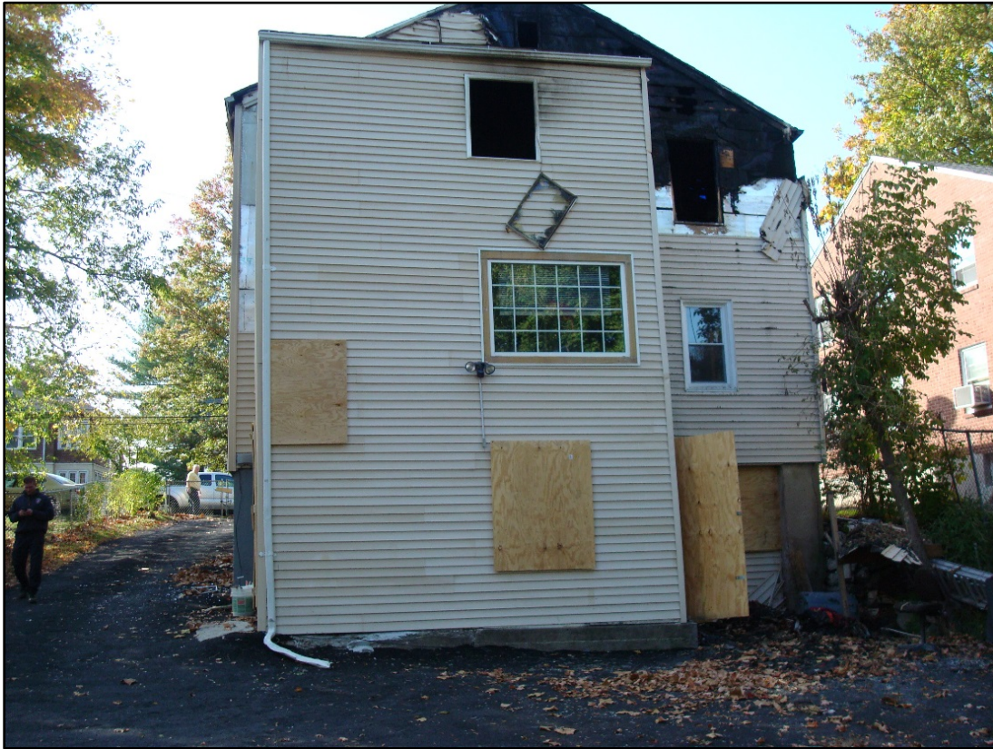
Photo 3. Side Charlie of the structure. An unoccupied apartment was in the basement. The entrance to the basement apartment is on the Bravo/Charlie corner.
