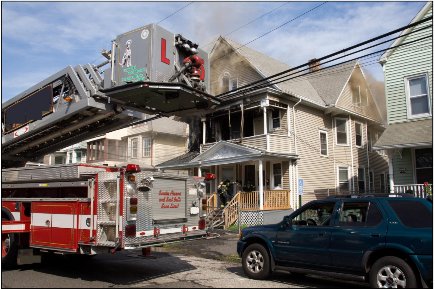
Photo 4. Conditions observed at 1608 hours by an off-duty fire fighter. Note: Smoke had changed to gray and brown in color and was emitting from the eaves and A- and D-side windows which were manually opened by personnel working on the 3 rd floor. A hoseline was being stretched to the 3 rd floor.
