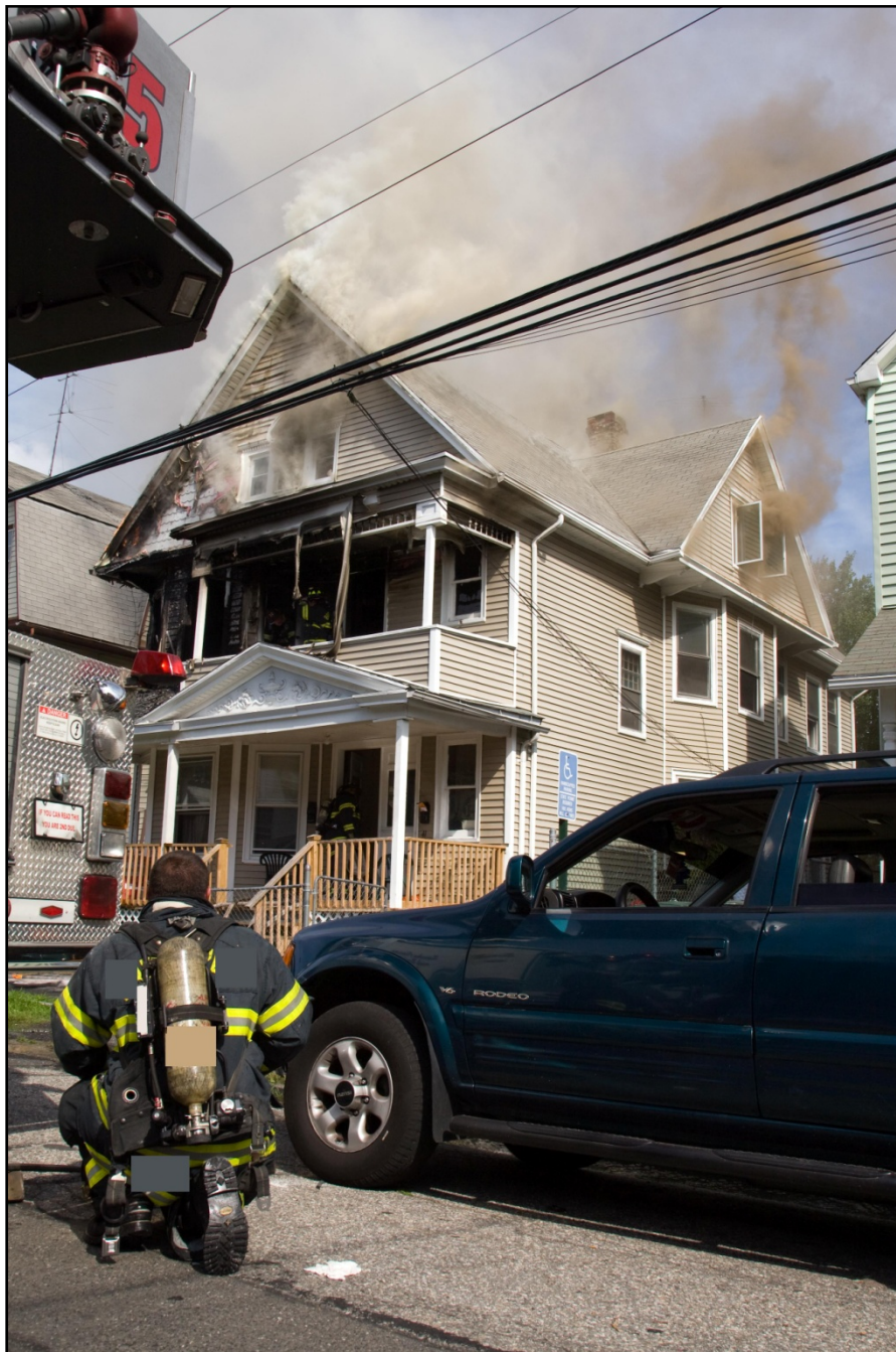
Photo 8. Conditions at approximately 1616 hours. Note: View from the A/D corner, scene conditions very close to when FF2 discovered FF1 pulling Victim #1 off the 3 rd floor stairs. White and gray smoke can be seen flowing from the A-side window and eaves while brown smoke flowed from the D-side window.
