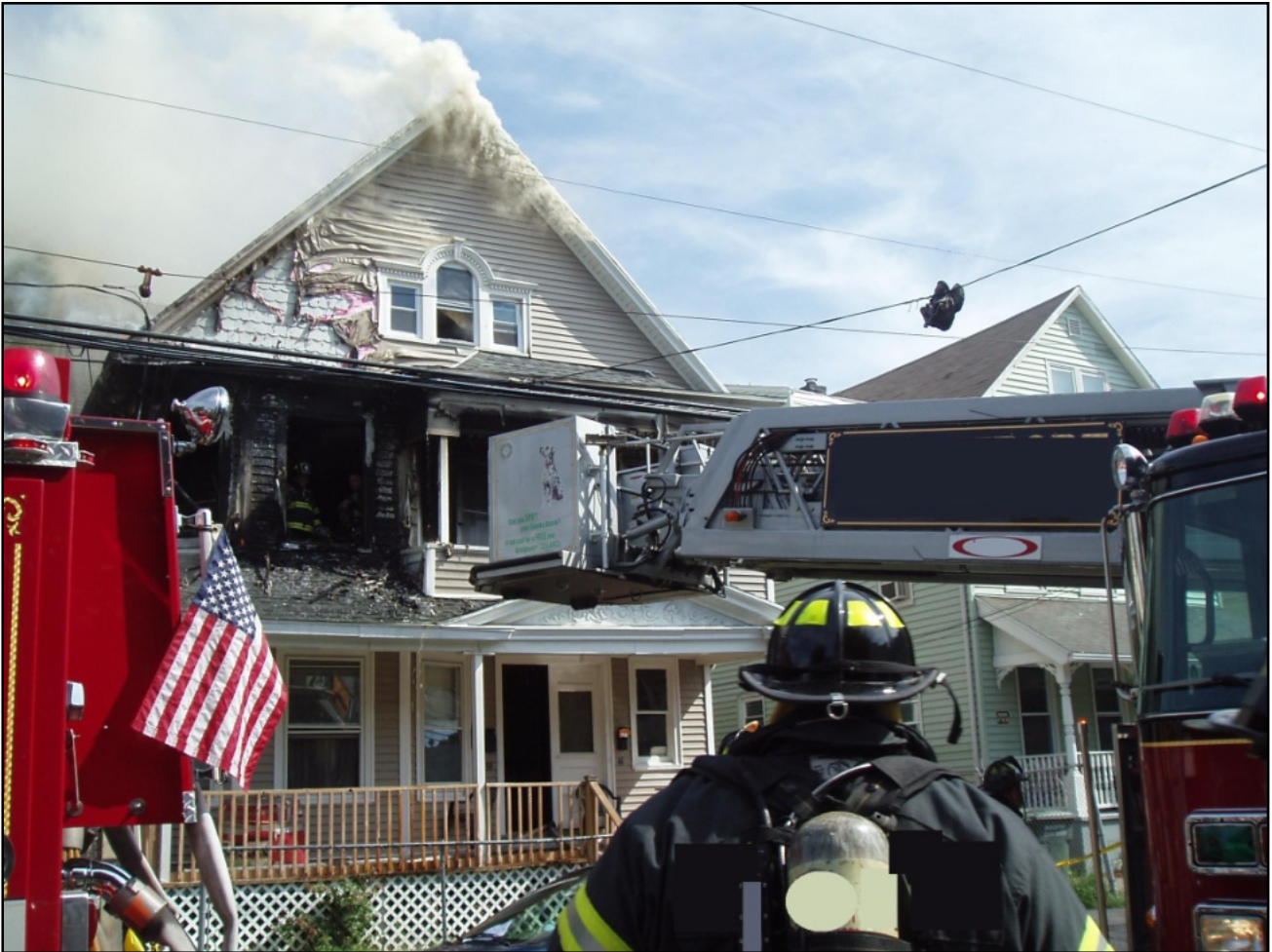
Photo 3. Initial conditions observed when the BC arrived on scene at approximately 1551 hours. Note: Fire was under control on the 2 nd floor and fire fighters were checking for extension. White-to-gray smoke can be seen flowing in the direction of right to left from the gables. The A-side window on the 3 rd floor had been opened for ventilation (unsure at what stage of the fire or by whom). (Photo courtesy of fire department.)
