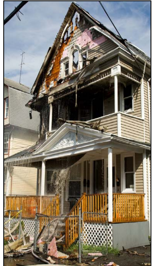
Incident structure following extinguishment. (Photo courtesy of Keith Muratori.)
