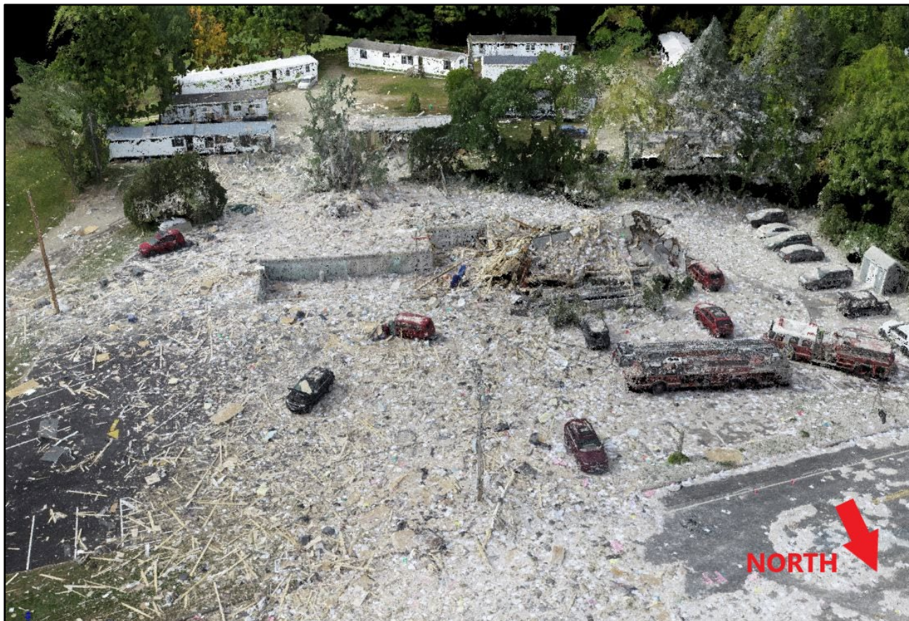
Photo 3. Drone footage of the office building and surrounding area after the explosion. A mobile home park was located to the south of the building property. (Photo courtesy of the Maine Office of the State Fire Marshal)
