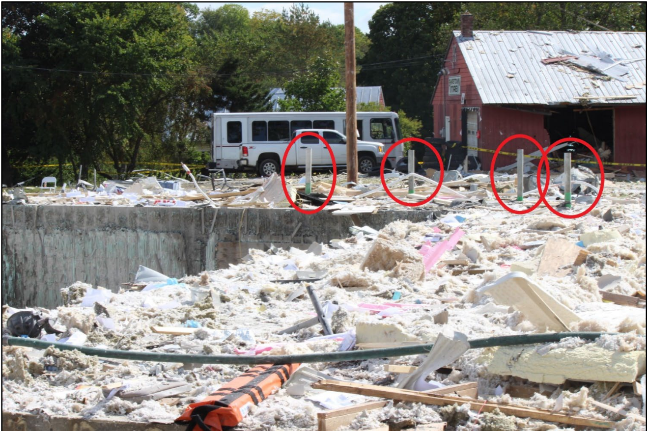
Photo 2. The bollards (red circles) that were placed to protect the air conditioning units in the parking lot on Side Bravo of the office building. When the bollards were driven into the ground, one of the bollards severed the propane supply line.
