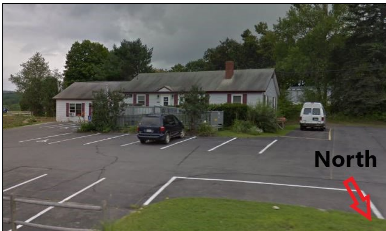
Photo 1. The original structure that was purchased in 2003 and before the renovation project in 2018.
