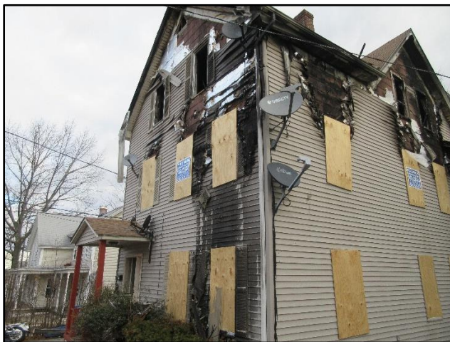
Photo 1. Side Alpha and Side Delta of the structure. NIOSH Photo
