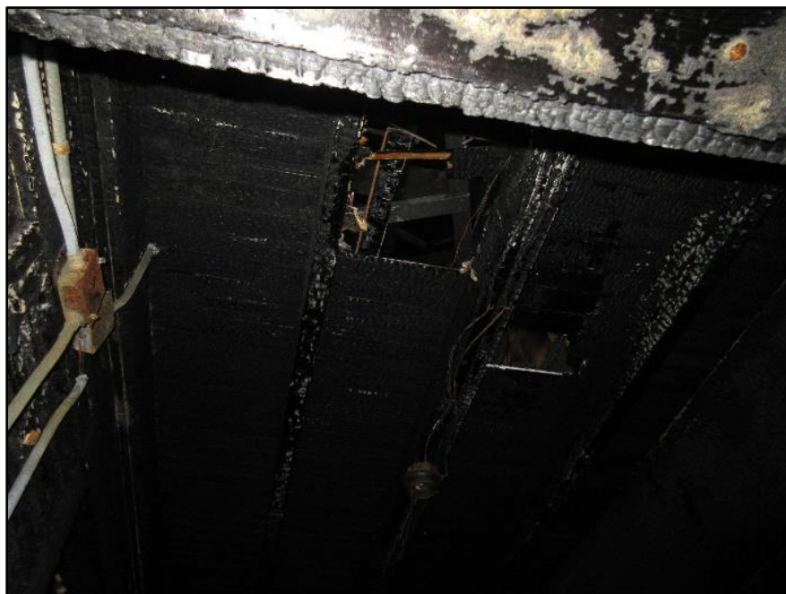
Photo 11. Holes in 3 rd floor porch shown from 2 nd floor. NIOSH Photo
