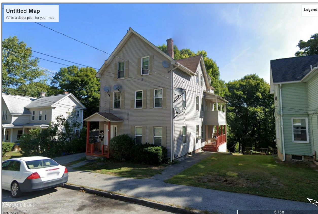
Photo 5. The fire building. There was access to all three floors by Side Alpha and Side Delta stairs. (Courtesy of Google Earth)
