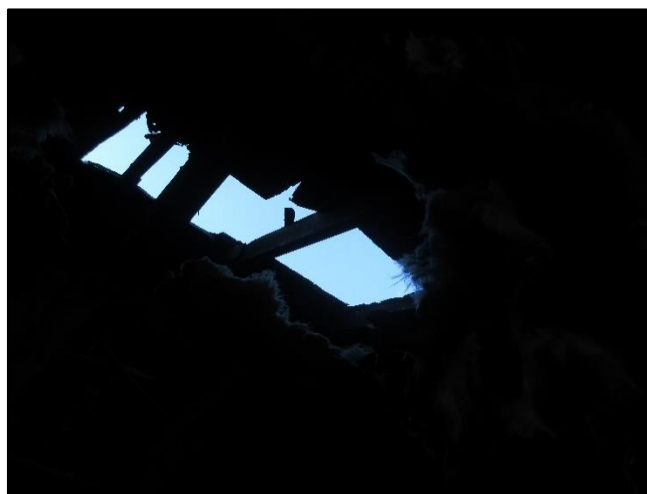
Photo 7. Roof vented by Ladder 3 on Side Bravo. NIOSH Photo
