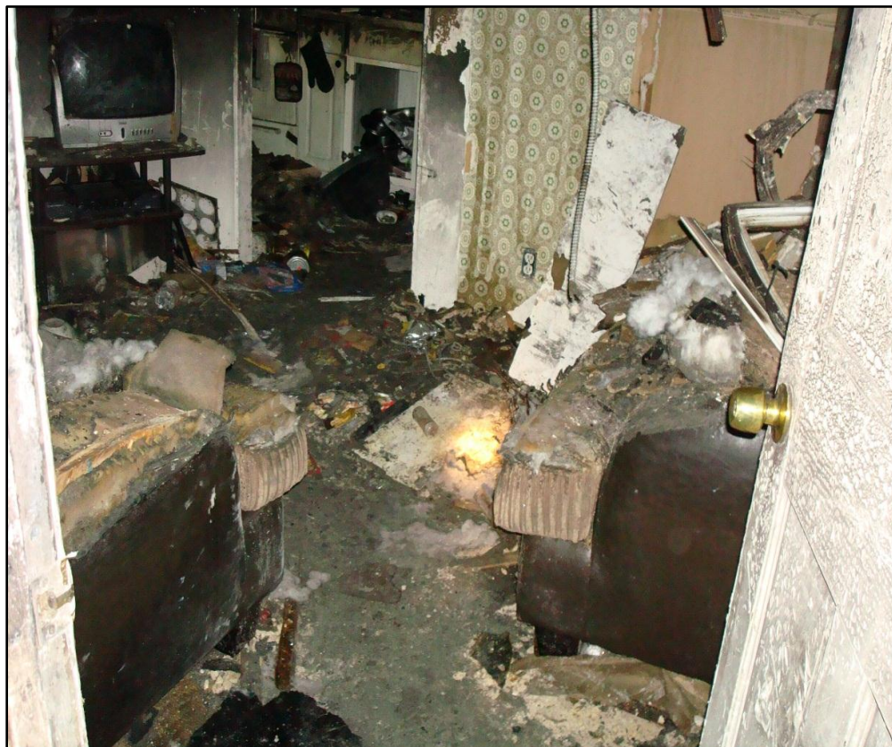
Photo 4. A view of the living room of the fire apartment from the doorway. The location of the two couches created ingress and egress problems for fire fighters. The victim was found in the kitchen near the entrance to the 2 nd bedroom
