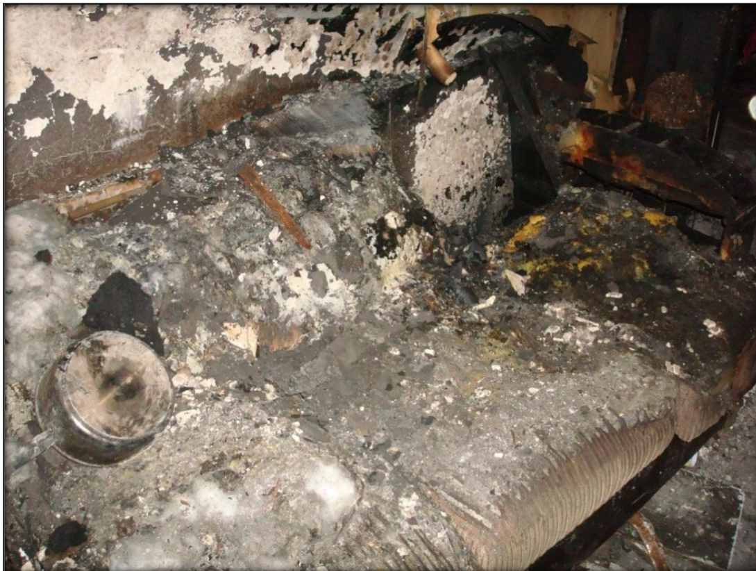
Photo 2. The pan that the female occupant used to attempt to extinguish the fire in the bedroom. The couch is located on the wall against the stairwell.
